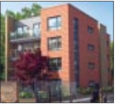
Gill Street, Limehouse, London E14 - ready in March 2009
