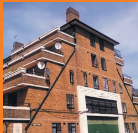
Lennox House in Hackney
