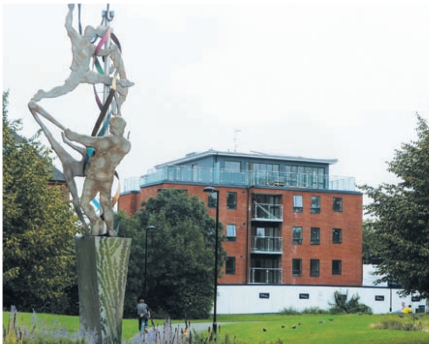
Ducere House, Viaduct Street, E2 0BZ
